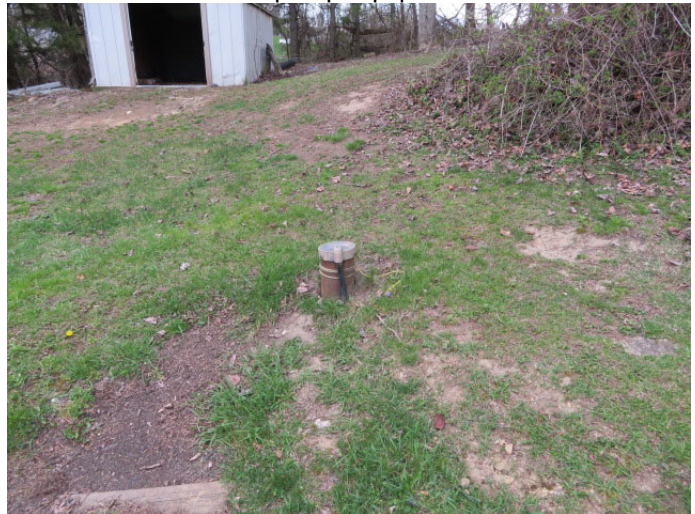
Above ground well head cover.
