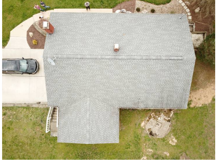
Aerial view of the roof structure
