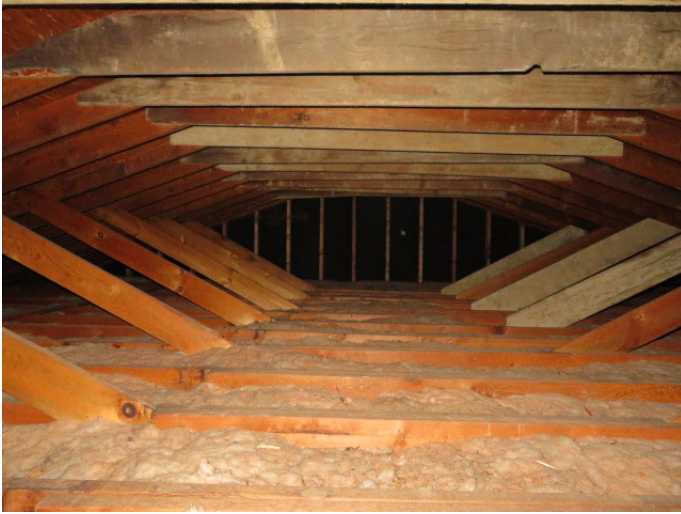
Reference photo of the attic structure.
